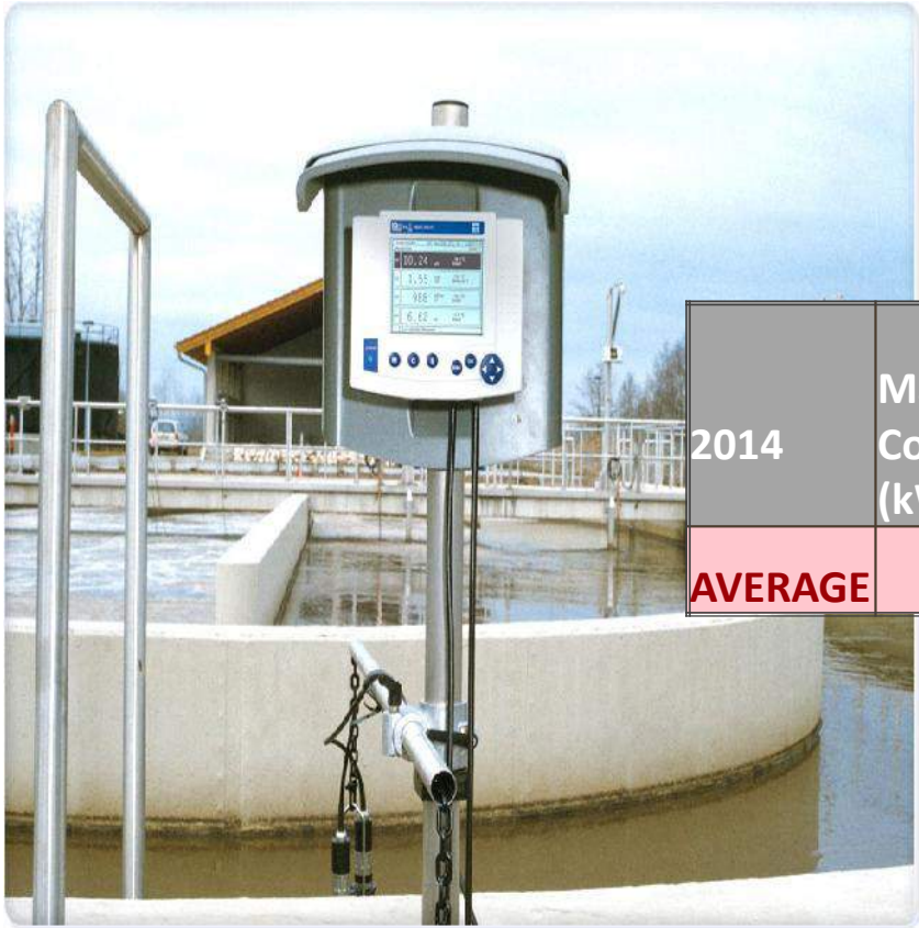
Auto-Aeration Control Mechanism
