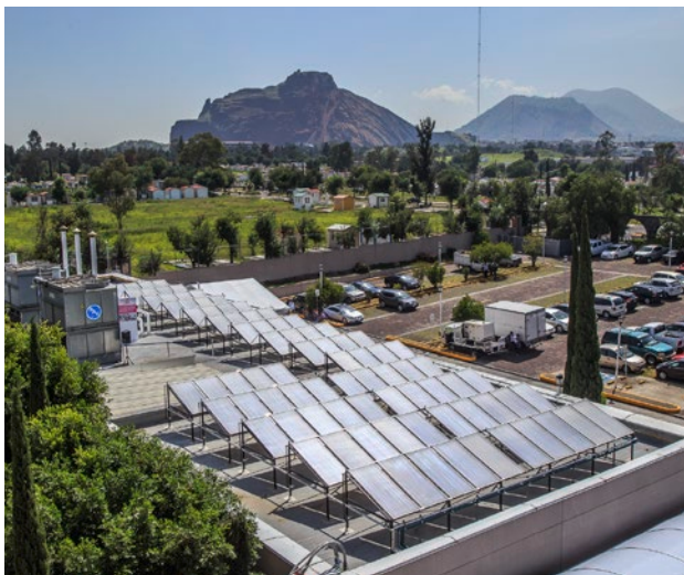
Solar Water Heaters installed on the rooftop of Public Building of Mexico City
