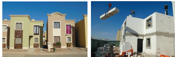
Images 1&2. New Housing NAMA in Hermosillo, Mexico (completed and under construction).
